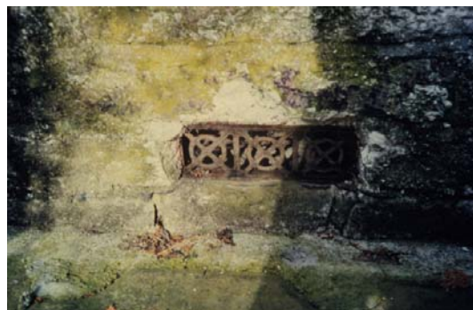
Obstructed underfloor vents
