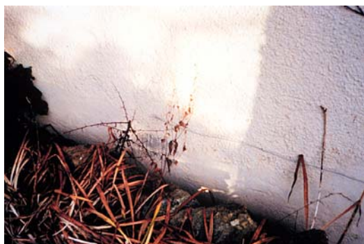
Obstructed underfloor vents
