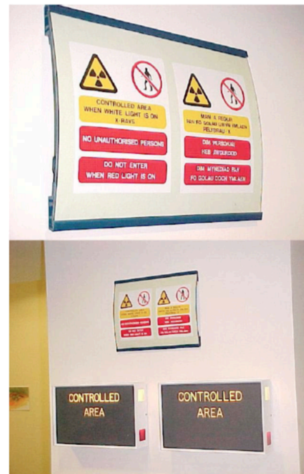
Figure A12.6 Safety signs and notices (in two languages) at the entrance to a radiotherapy bunker; the illuminated interlocked warning signals are shown in use in the lower image
